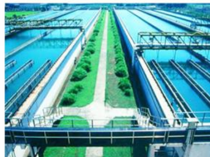
Drinking Water Plants & Distribution Networks
